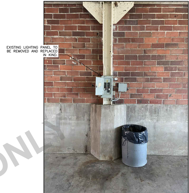
PORT BUILDING INTERIOR — LOOKING NORTH (6-3) NO SCALE
